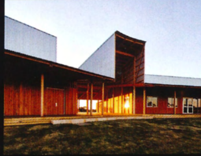
Pingelly Recreation and Cultural Centre iredale pedersen hook architects & Advanced Timber Concepts Studio AUSTRALIA
