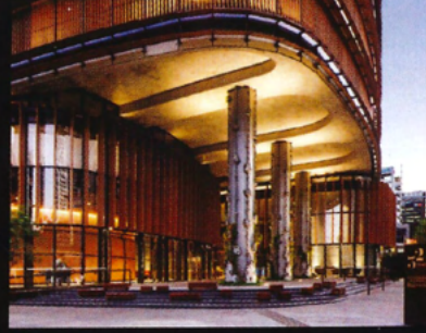
32 Smith Street Fender Katsalidis AUSTRALIA
