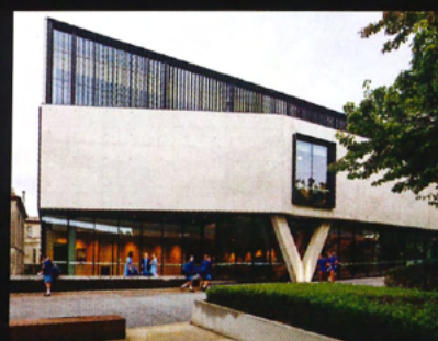
The Clendon Centre Architectus AUSTRALIA
