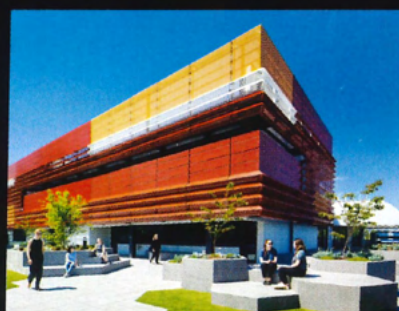
Port Melbourne Secondary College Billard Leece Partnership (BLP) AUSTRALIA
